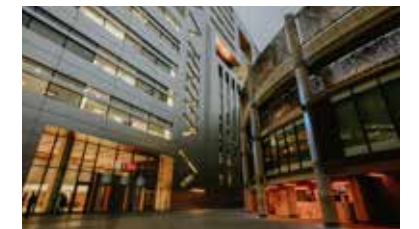
UBS Main Office
